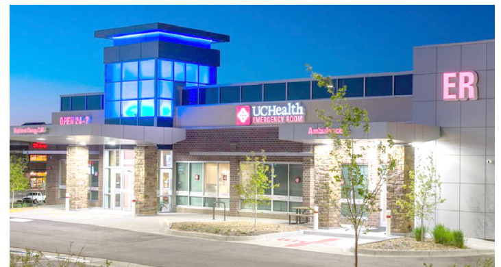
Preferred character for new office /medical services development focuses on attracting small tenants which provide local services
