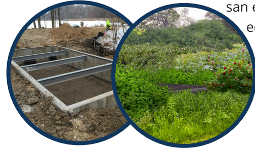
[Far left] The chamber that will hold the spent-lime material. [Left] A rendering of what the completed system will look like.
