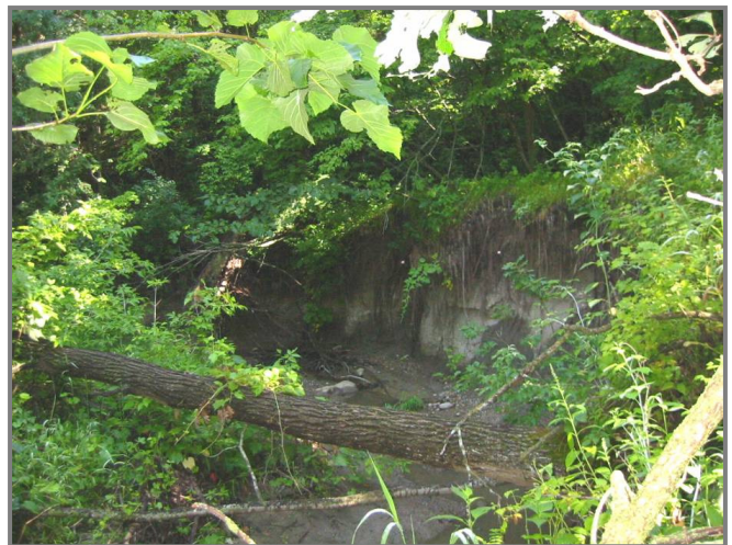
Figure 38 Severe bank erosion is found in the 400-foot reach of Bluff Creek at Site 20. Flow causes and determines the degree of streambank erosion in Bluff Creek.
