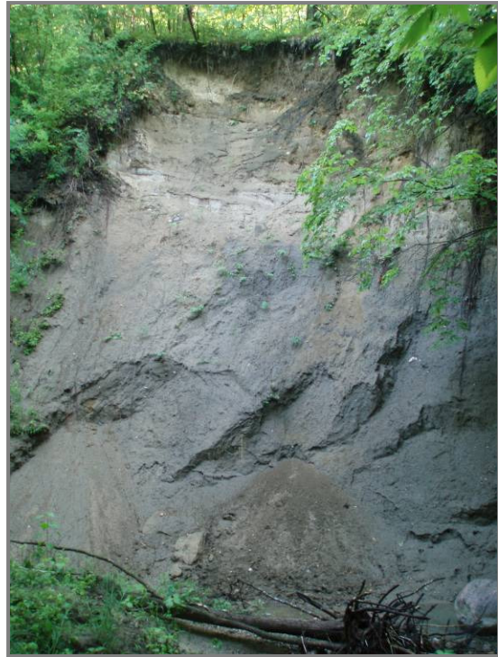
Figure 37 Site 11 noted slope failure immediately adjacent to the stream
