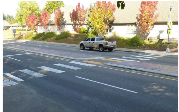
Example of median crossing island on a two-lane street (top) and on a four-lane street with a pedestrian crossing beacon (bottom).
