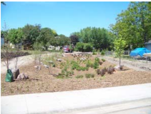
Raingarden on Laredo Drive Source: City of Chanhassen
